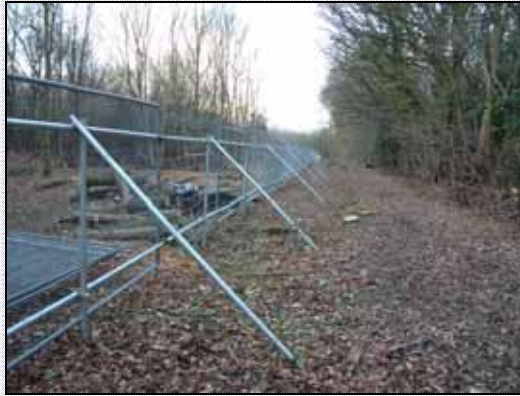
Heras fencing wired to scaffold braced posts
