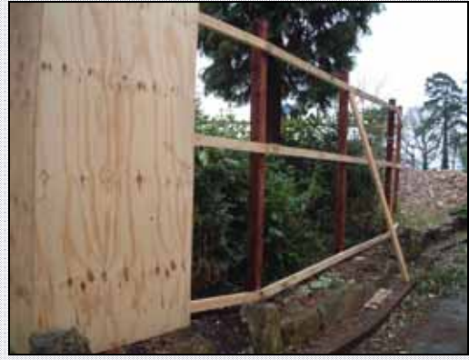
Board specification on secure wooden posts
